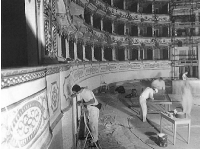
Figure 4. Detail of the wall restoration in the cavea.
