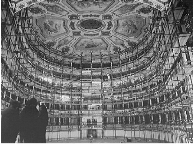
Figure 3. Scaffolding inside the theatre during the refurbishment.
